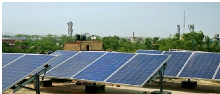
Solar panels were installed at our Delhi office in India.
